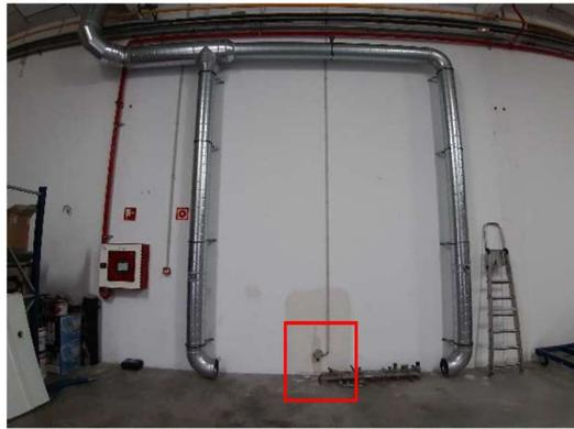
Figure 3. Leak detection sensor and location in Charging zone prepared with the air extraction system.
